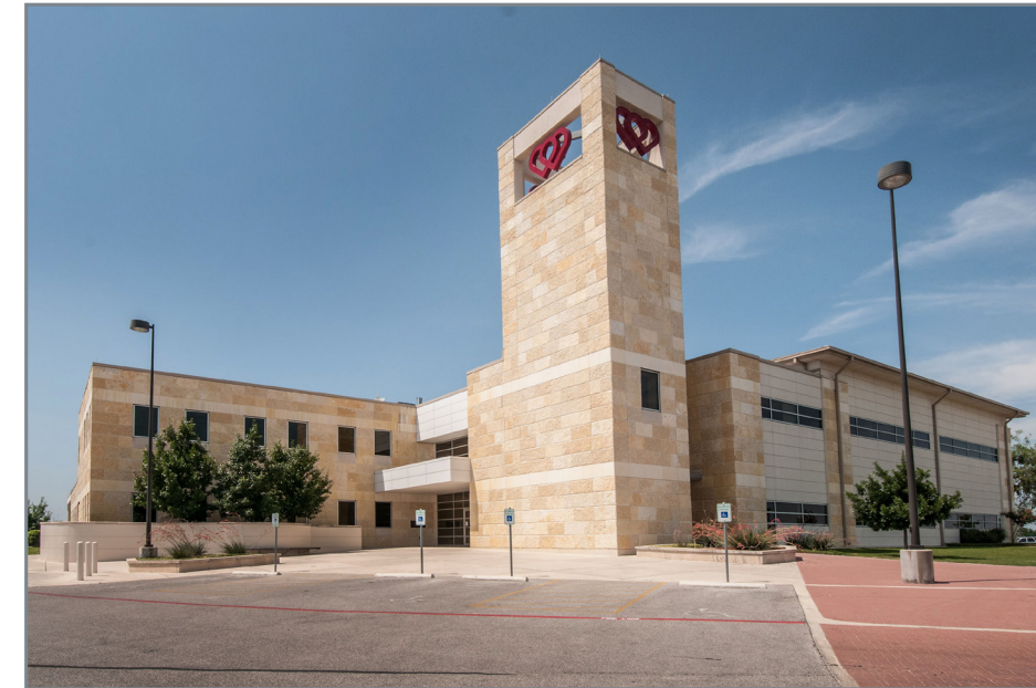
Heavily regulated organizations like BioBridge Global must have easy access to metrics to monitor the overall health of the Quality System.
